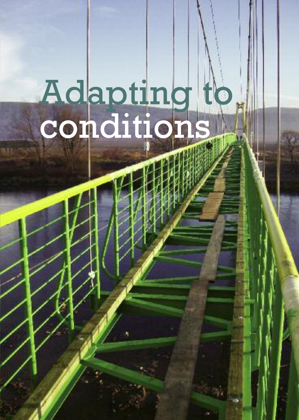
FOOTBRIDGE, WITRYLOW, POLAND
