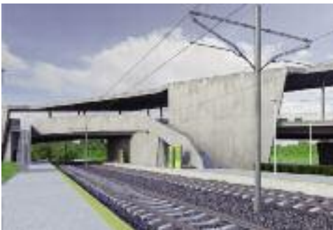
RAILWAY VIADUCT, WROCLAW, POLAND
