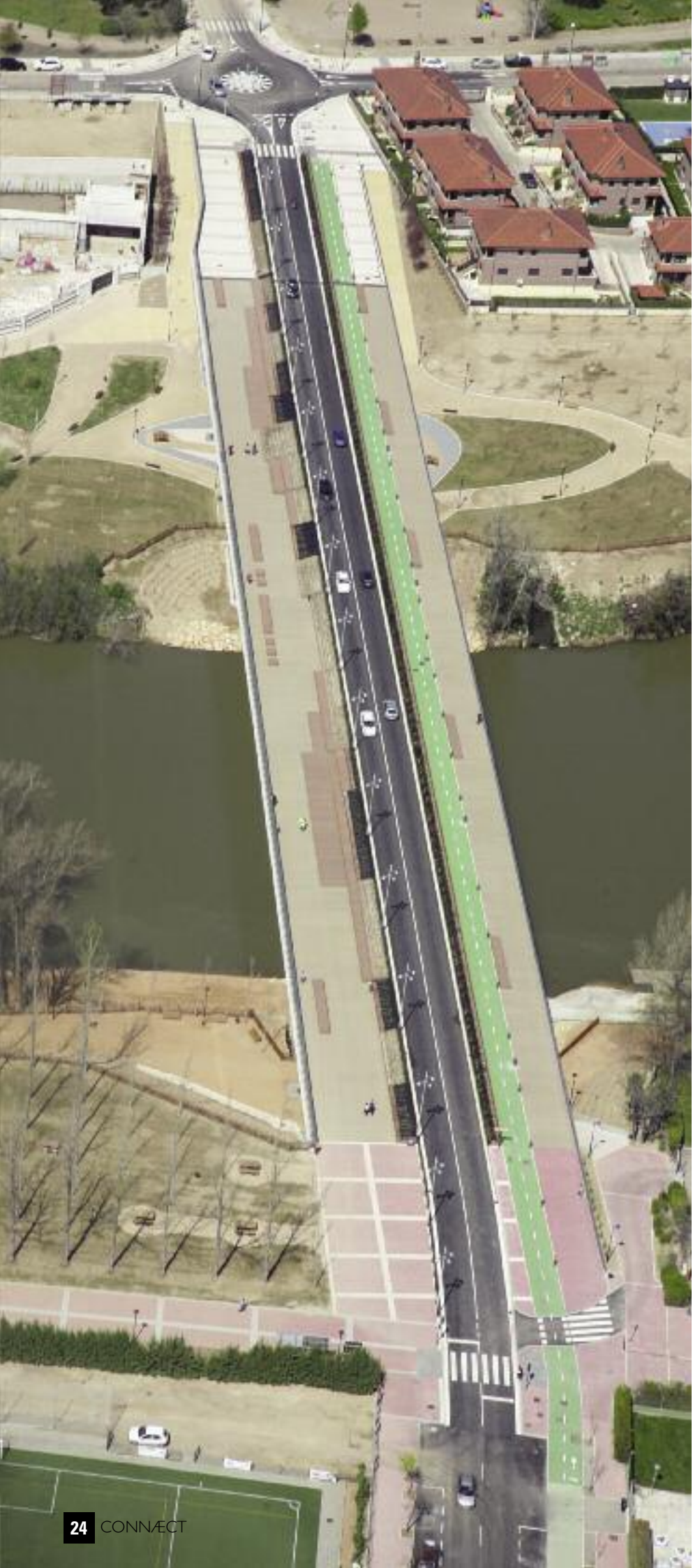
PISUERGA RIVER BRIDGE, VALLADOLID, SPAIN
