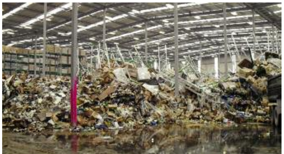
Post-tensioned warehouse floors remained intact, providing a solid base for the clean-up of collapsed racking, and businesses were quickly able to resume trading.
