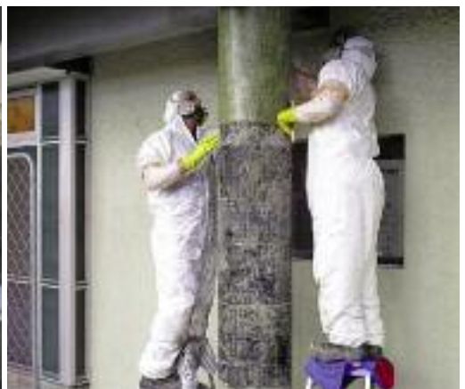
Just five days before the September earthquake, BBR completed the strengthening of 23 circular columns at the University of Canterbury's Student Services Building.
