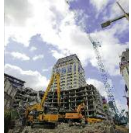
Demolition underway of the car park of the Hotel Grand Chancellor – giving an insight into the scale of work necessary.
