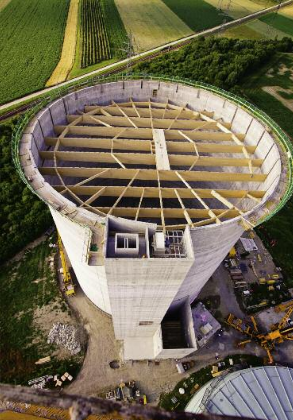
SUGAR SILO, TULLN, AUSTRIA
