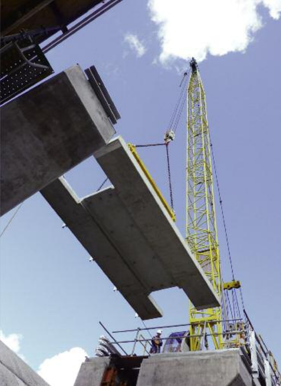
WELLINGTON DAM, COLLIE, WESTERN AUSTRALIA
