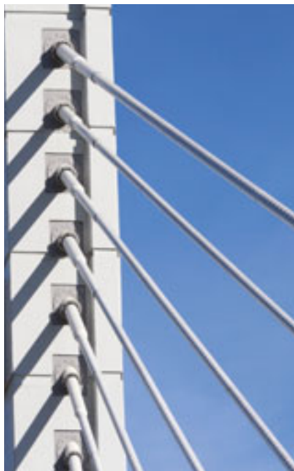
1 BBR HiAm CONA stay cables anchored at a pylon.
