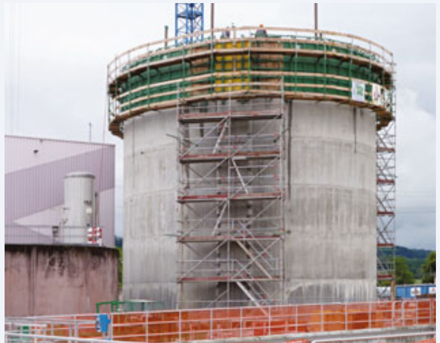
1 The new 15.8m high wastewater tank at ARA Reinach takes shape.
