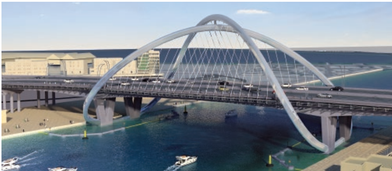
Visualization of the new Infinity Bridge in Dubai which features a 42m high arch, shaped like the mathematical symbol for infinity.
