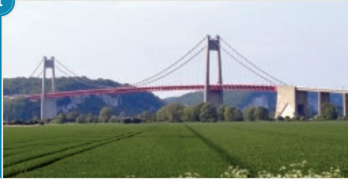
1955 – Tancarville Bridge, Seine-Maritime, France: Constructed in the late 1950s, this landmark project featured 120 BBRV rock anchors which were installed to secure the huge concrete block where the bridge's suspension cables are also anchored.
