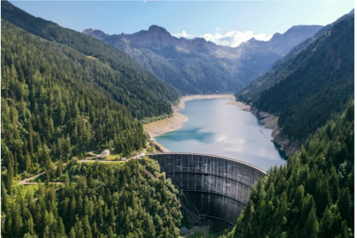
Frera Dam, Lombardy, Italy: Consolidation work required 53 BBRV anchors to be installed deeply into the rock on the left side of the dam.
