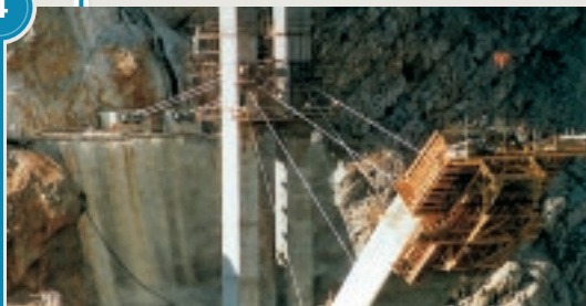
1990s – Maslenica Bridge, Croatia: BBRV ground anchors were used to secure the temporary stay cables to the rock face during construction of this arch bridge.
