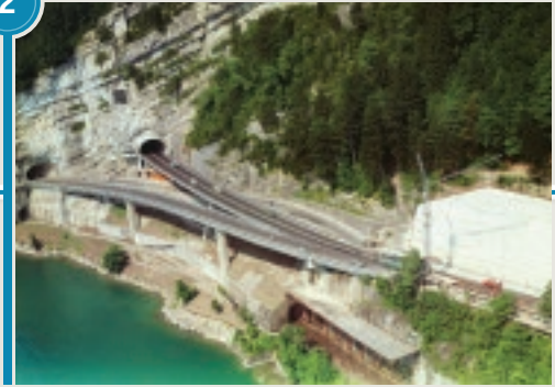
1960s – Axenstrasse near Brunnen/Mositunnel, Switzerland: Seven BBRV ground anchors were used to support the new viaduct where the Axenstrasse joins the A4 motorway after it emerges from the Mositunnel. Image courtesy of ETH-Bibliothek Zürich, Bildarchiv, Photographer: Comet Photo AG (Zürich), Reference: Com_F65-05257, licensed under CC BY-SA 4.0.
