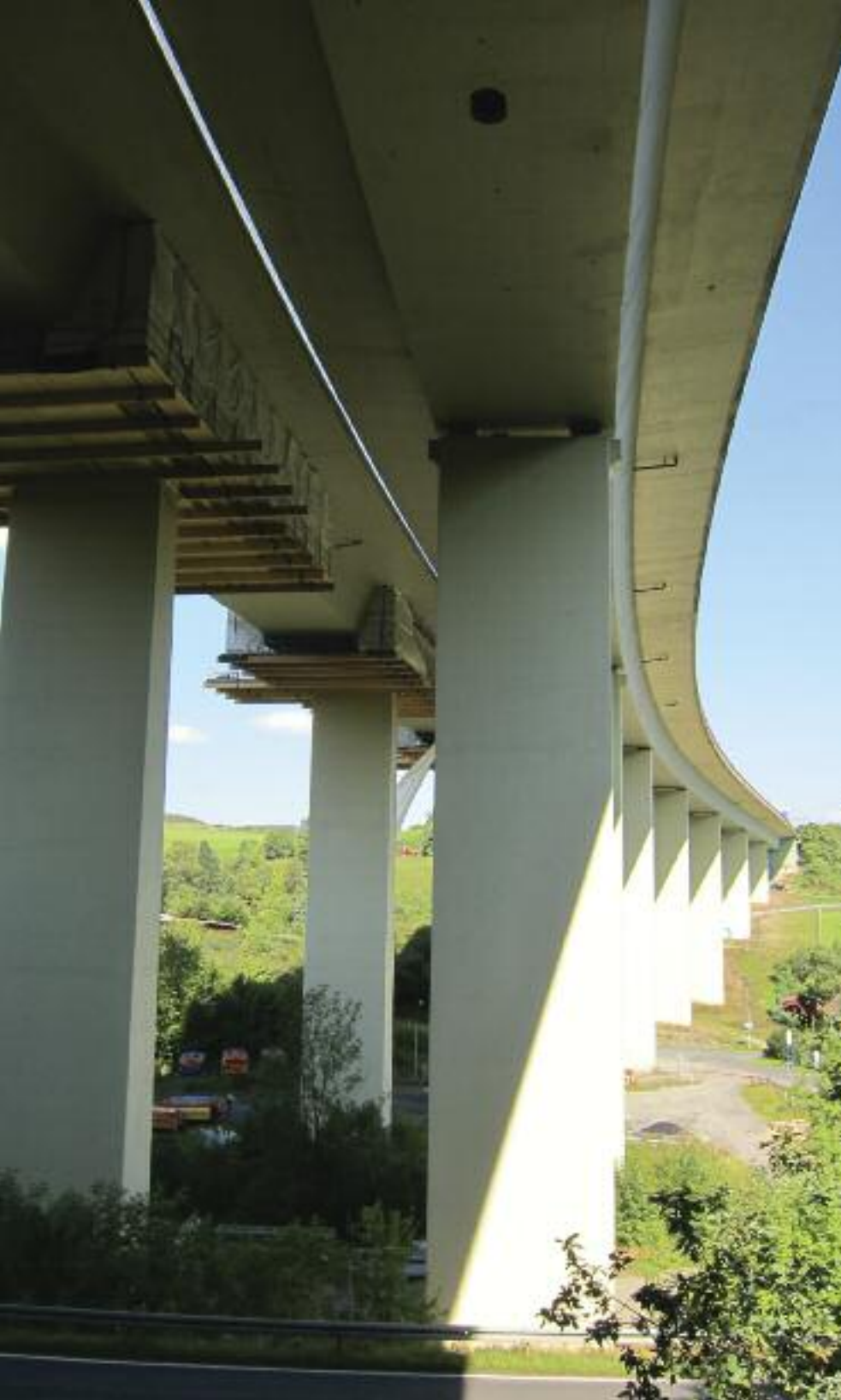
EMERGENCY REPAIRS, A45 MOTORWAY, GERMANY
