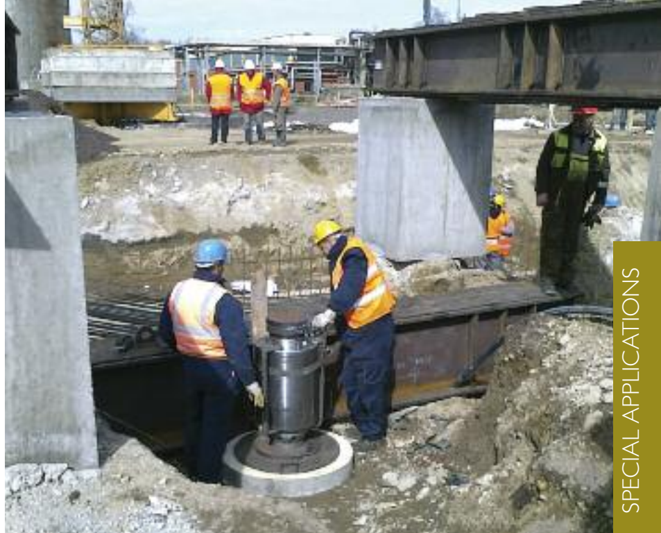
COMBINED HEAT & POWER PLANT, SISAK, CROATIA
