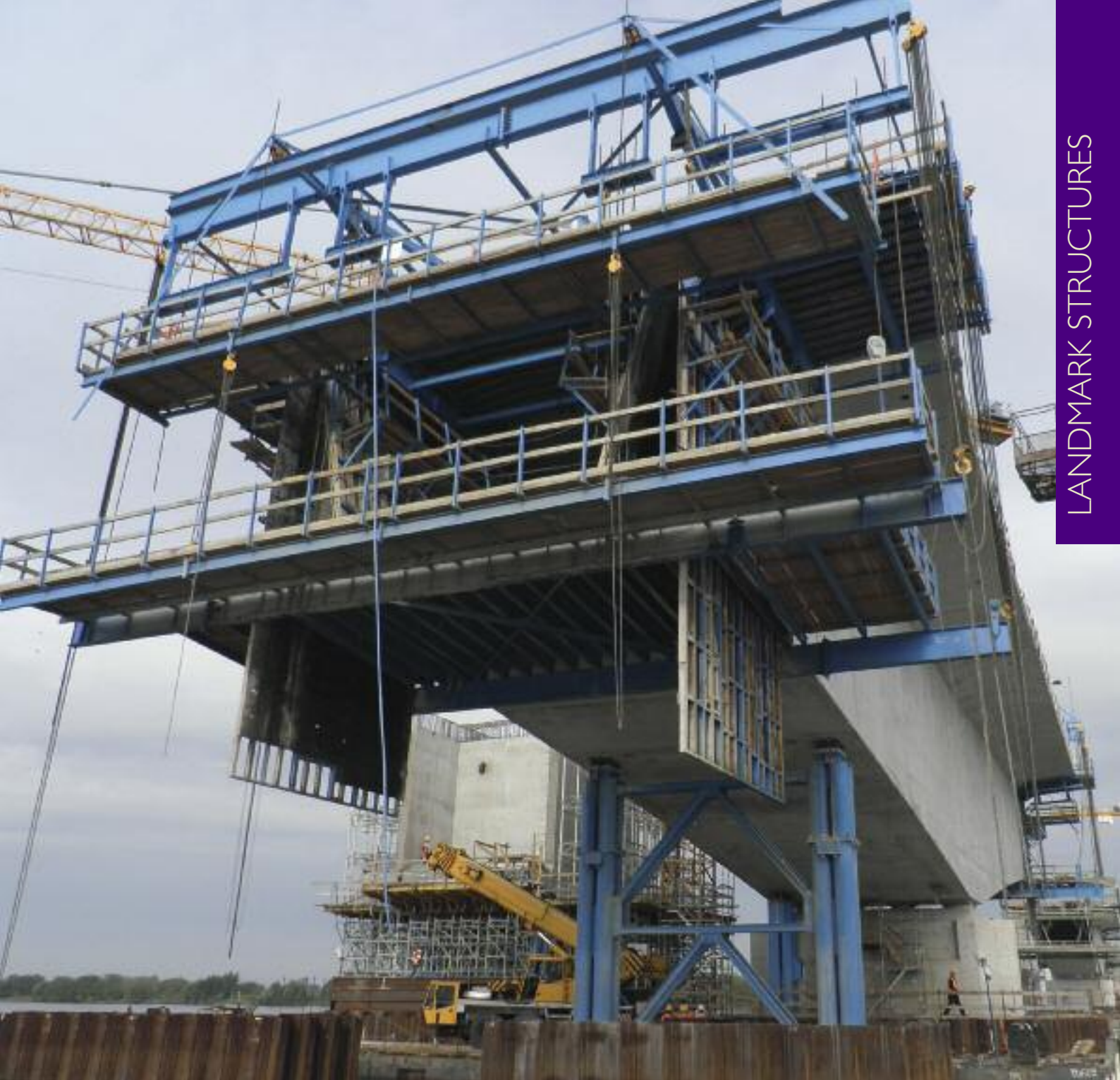
BBR BALANCED CANTILEVER CONSTRUCTION
