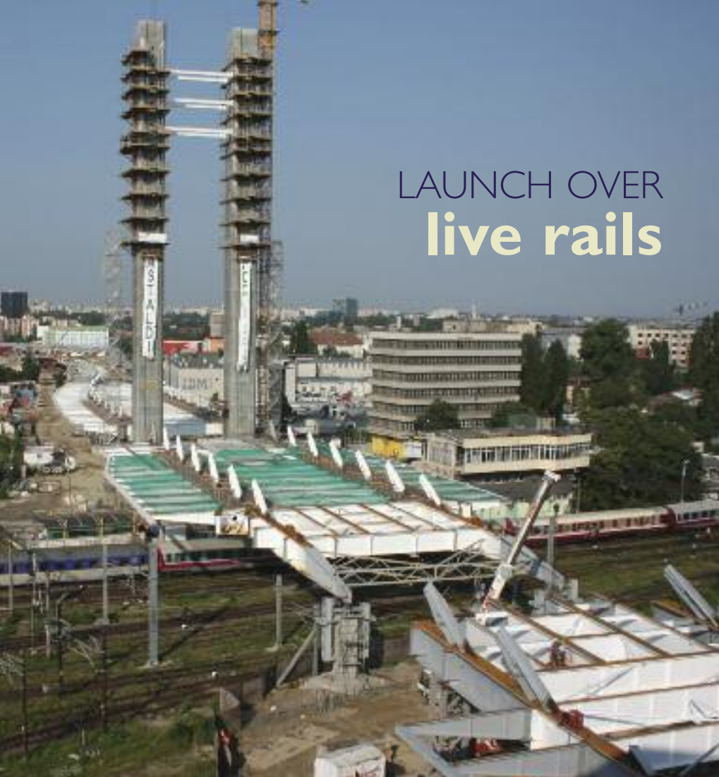
BASARAB OVERPASS, BUCHAREST, ROMANIA
