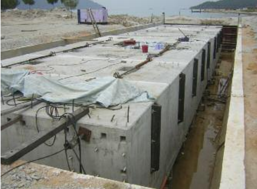
SEGMENTAL PONTOON, LUMUT PORT, PERAK, MALAYSIA
