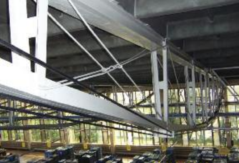
FACTORY ROOF STRENGTHENING, PABIANICE, POLAND
