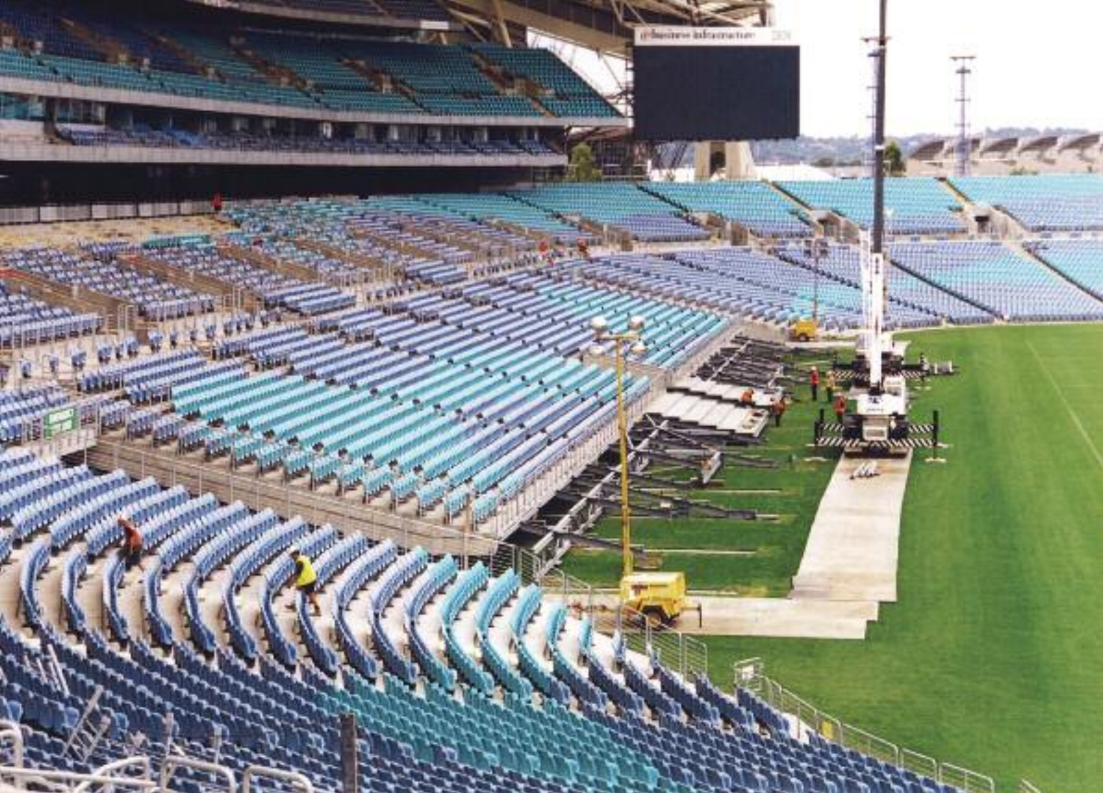
STADIUM AUSTRALIA RECONFIGURATION, HOMEBUSH, NEW SOUTH WALES, AUSTRALIA
