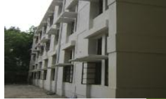
SEISMIC RETROFITTING OF SCHOOL, NEW DELHI, INDIA
