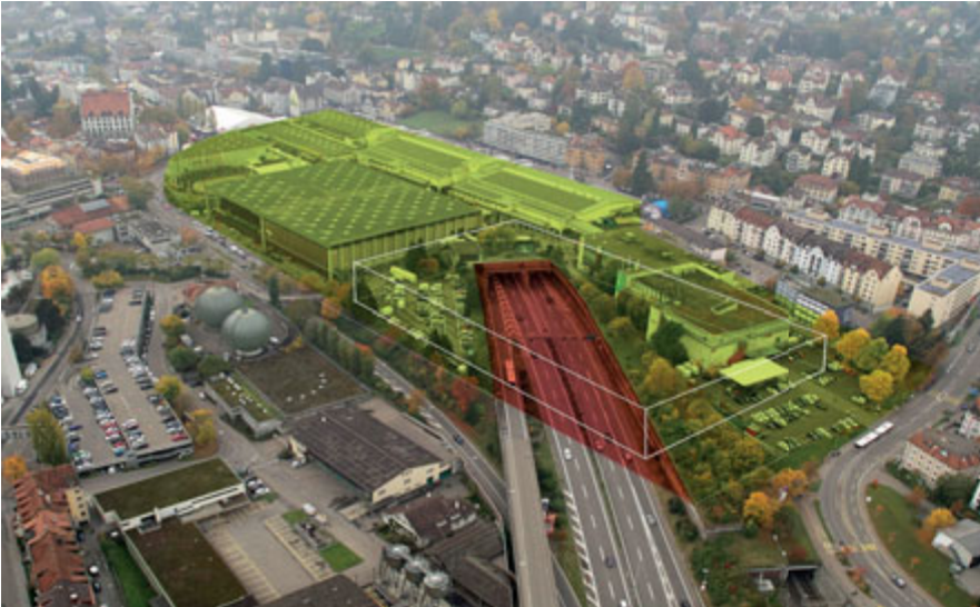
A 180m long roof over the Rosenberg Tunnel was needed to form part of the base for the new Hall 1 of the Olma Messen exhibition complex. Image courtesy of Olma Messen.
