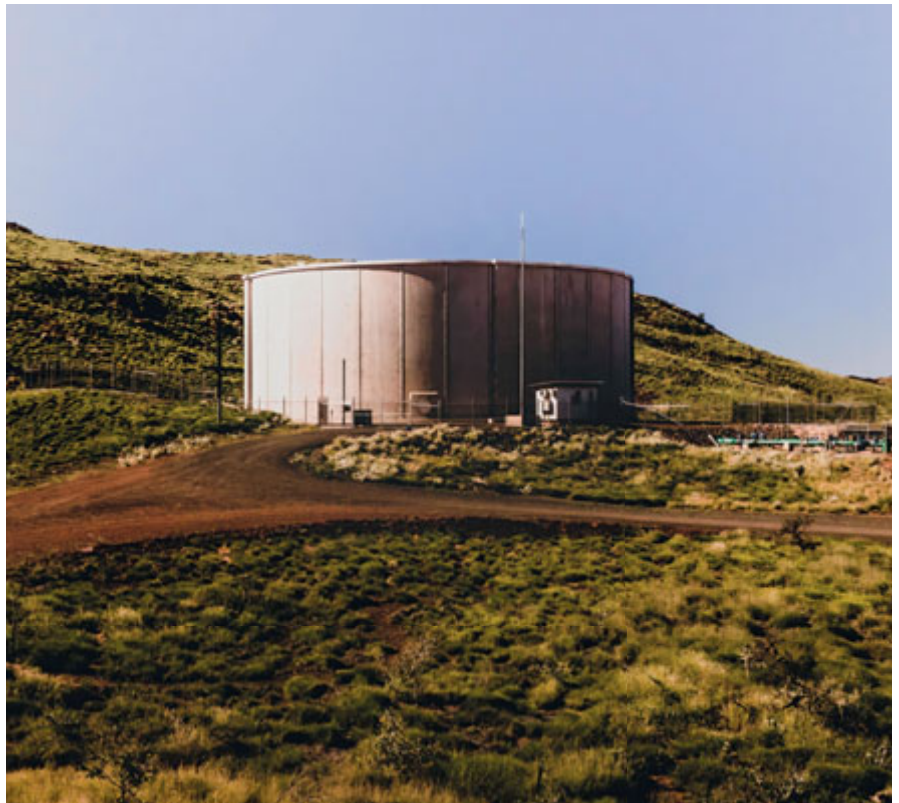
The new 42m diameter water tank in Karratha was designed and constructed of post-tensioned precast concrete panels.
