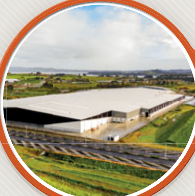
Foodstuffs Distribution Centre, Auckland – where BBR Contech installed the latest CONA CMF flat post-tensioning technology to create a 74,000m 2 floor slab – the largest ever to be constructed in a single project in New Zealand.
