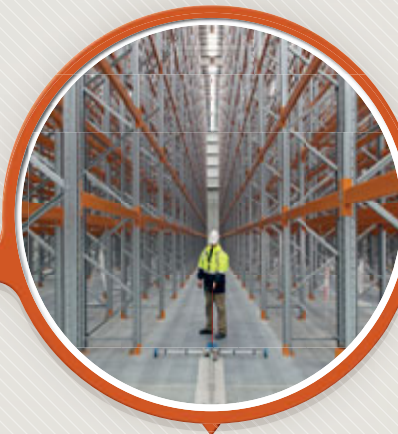
James Pascoe Group Distribution Centre, East Tamaki – this 25,000m 2 award-winning VNA (Very Narrow Aisle) super-flat PT floor was constructed by Conslab, with specialist PT expertise from BBR Contech who helped to deliver the best floor flatness level in the world.
