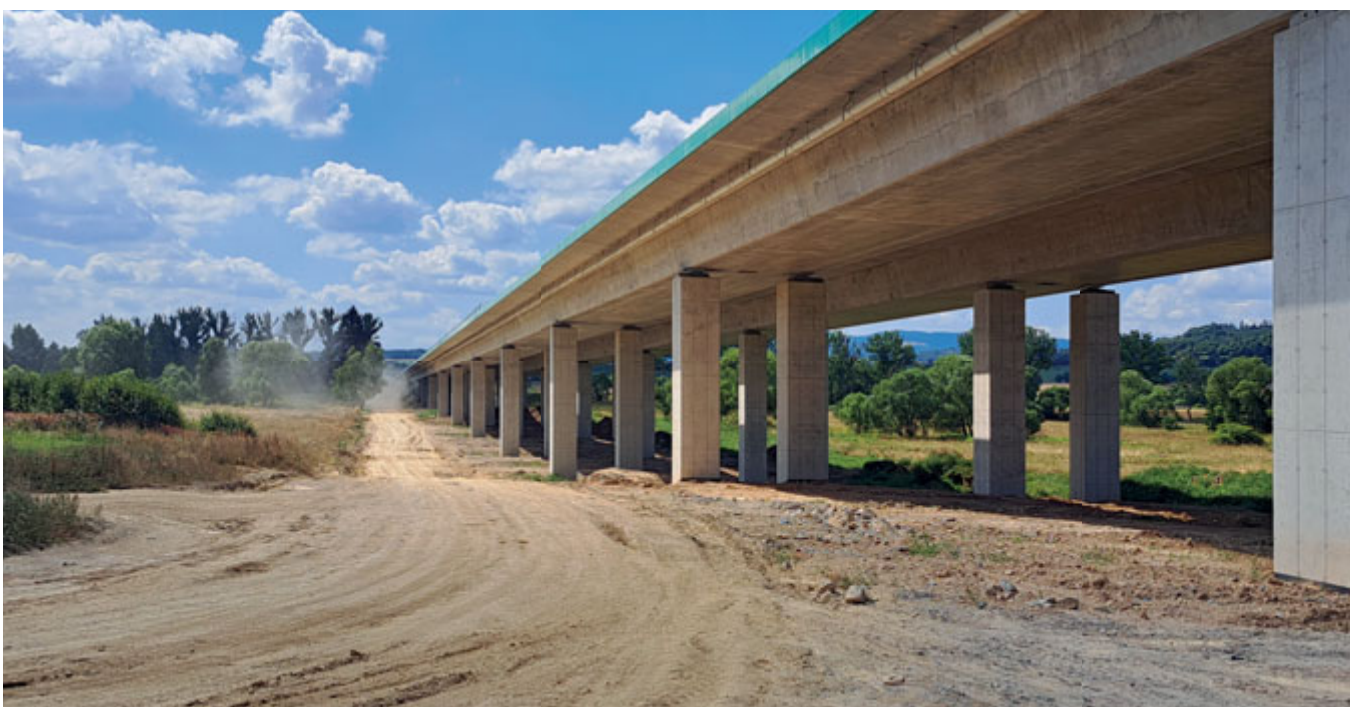
Flyover structure WS-54 after launching.
