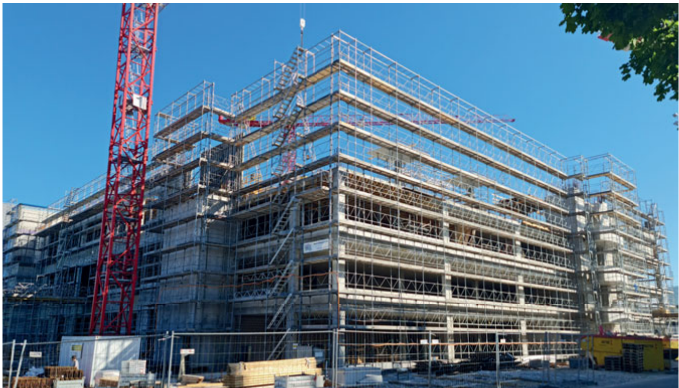
Overview of the building façade while work was in progress.
