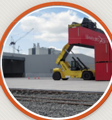
Fonterra, Darfield – this is probably the largest development to use post-tensioned slabs on one site. To date, a total of 80,900m 2 of PT slabs have been constructed for drystore warehousing, packing stores, coolstore and heavy-duty external pavements.
