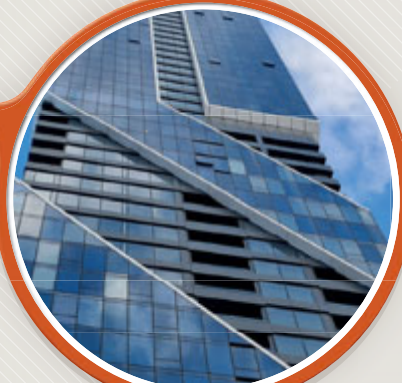
The Pacifica Building, Auckland – this stunning 57-floor mixed use tower is a new landmark on the Auckland skyline and was realized using BBR post-tensioning for the elevated floors and lateral load resisting system.
